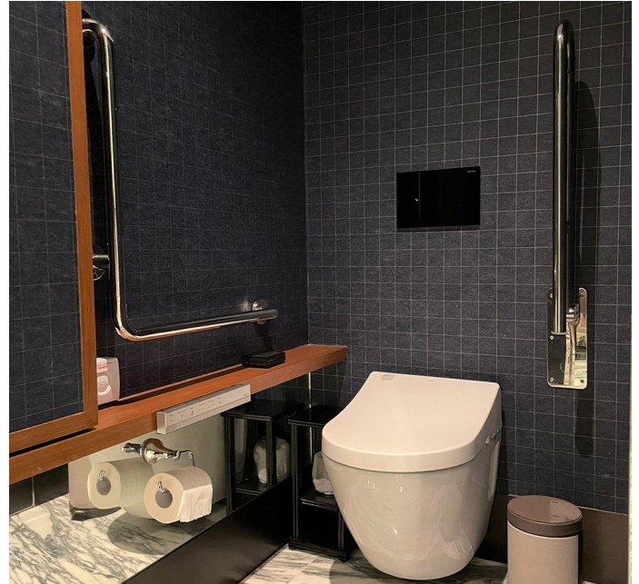
WC with handrails
